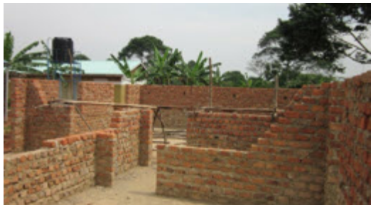
Maternity wing under construction
